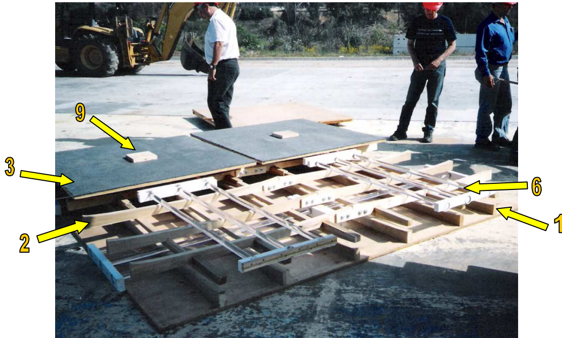
Figure 5. Four earthquake protectors in the process of assembly.
