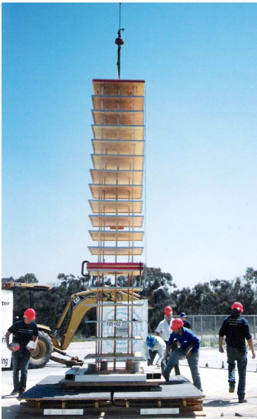
Figure 4. Building model erection.
